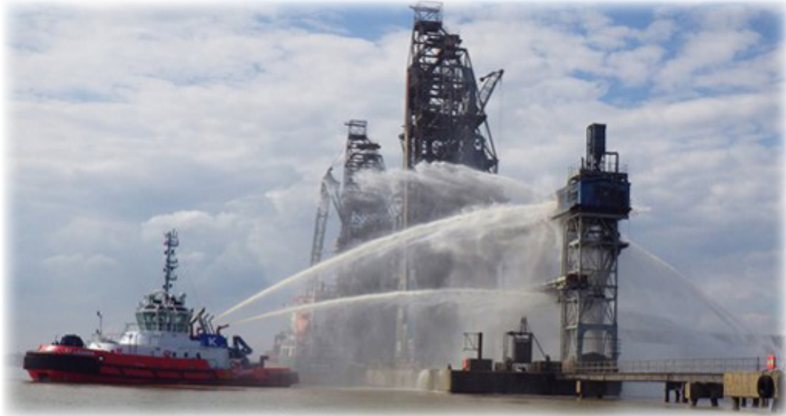
Image 1: Conveyor fire being extinguished
