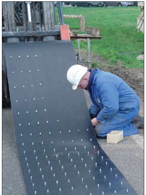
Preparing a belt for dragging into the elevator casing.
