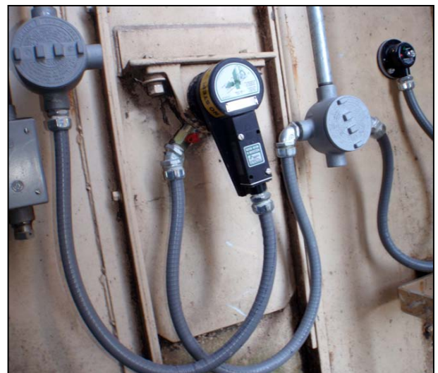
Whirligig on Bucket Elevator with M800 Elite Speed Switch
